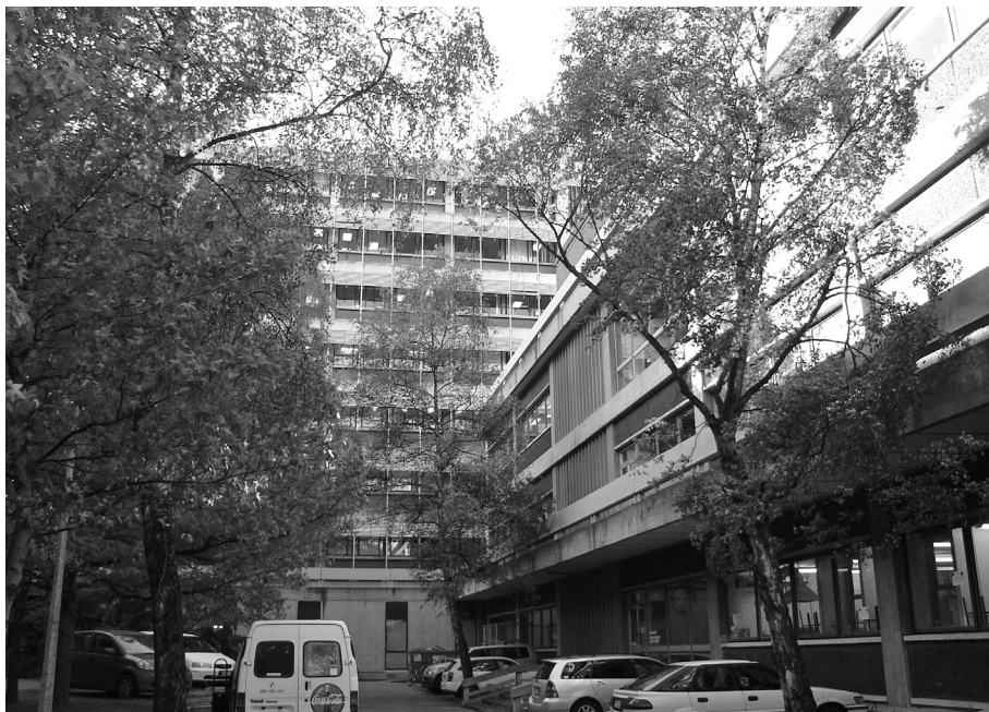
University of Otago Chemistry Building
