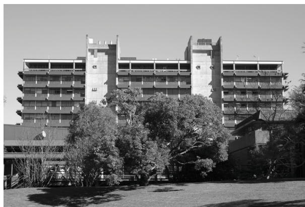
Chemistry Department building at Auckland University 2001. The grassy area is now the Kate Edger Information Commons.
