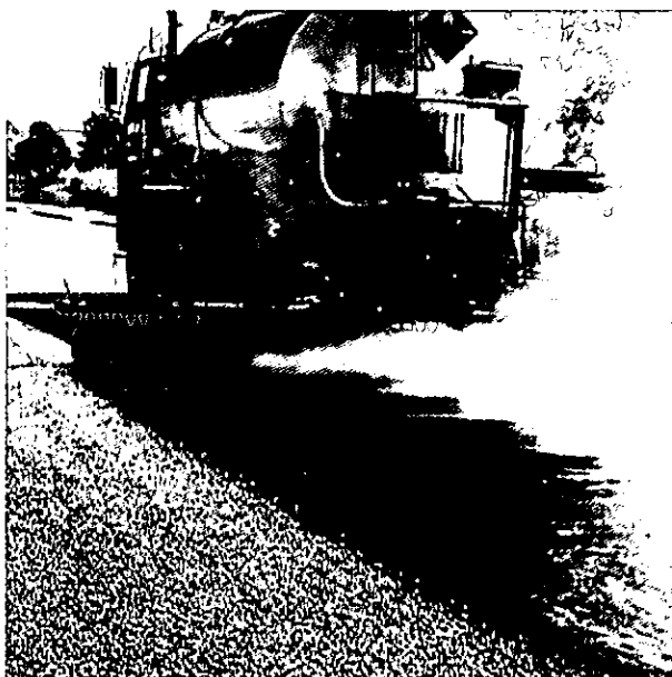
Figure 4: Spraying polymer modified bitumen on Carnegie Street in Napier.
