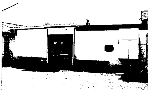
Above: West Block (1930s) and adjoining link-block (Offices, Library, Instrument Rooms).
